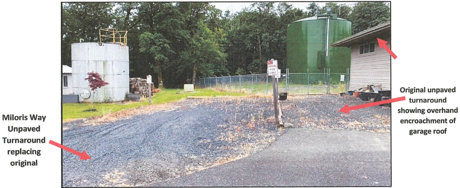
Photo 1. Miloris Way Unpaved Turnaround Photos taken June 30, 2022
