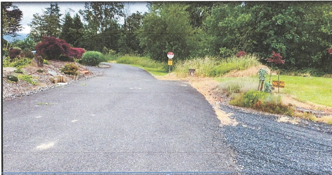
Photo 2. This is the end of Miloris Way paved to 20 ft wide. The photo shows the road reduces to 10 ft wide with two additional homes on that portion of Miloris Way.
